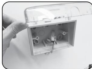
1. When installing the HYBOXWP ensure the product is mounted securely against the wall using the drill points in the covered recesses. Ensure the screw area is well sealed with silicone to protect the IP rating and apply internal screw caps.
